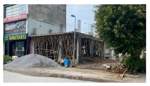
Figure 2: Conventional method of commercial building construction in Pakistan.
